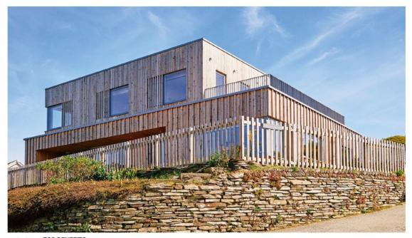
ECO BENEFIT'S Replacing a 1930s bungalow that was on the verge of collapse, this two-storey, four-bedroom home overlooks Cornwall's Mawgan Porth headland. Its owner wanted a house with good eco credentials, so Kast Architects created a highly insulated timber frame, forming an air-tight structure with low heating costs, and included photovoltaic (PV) panels on the roof to generate electricity.
