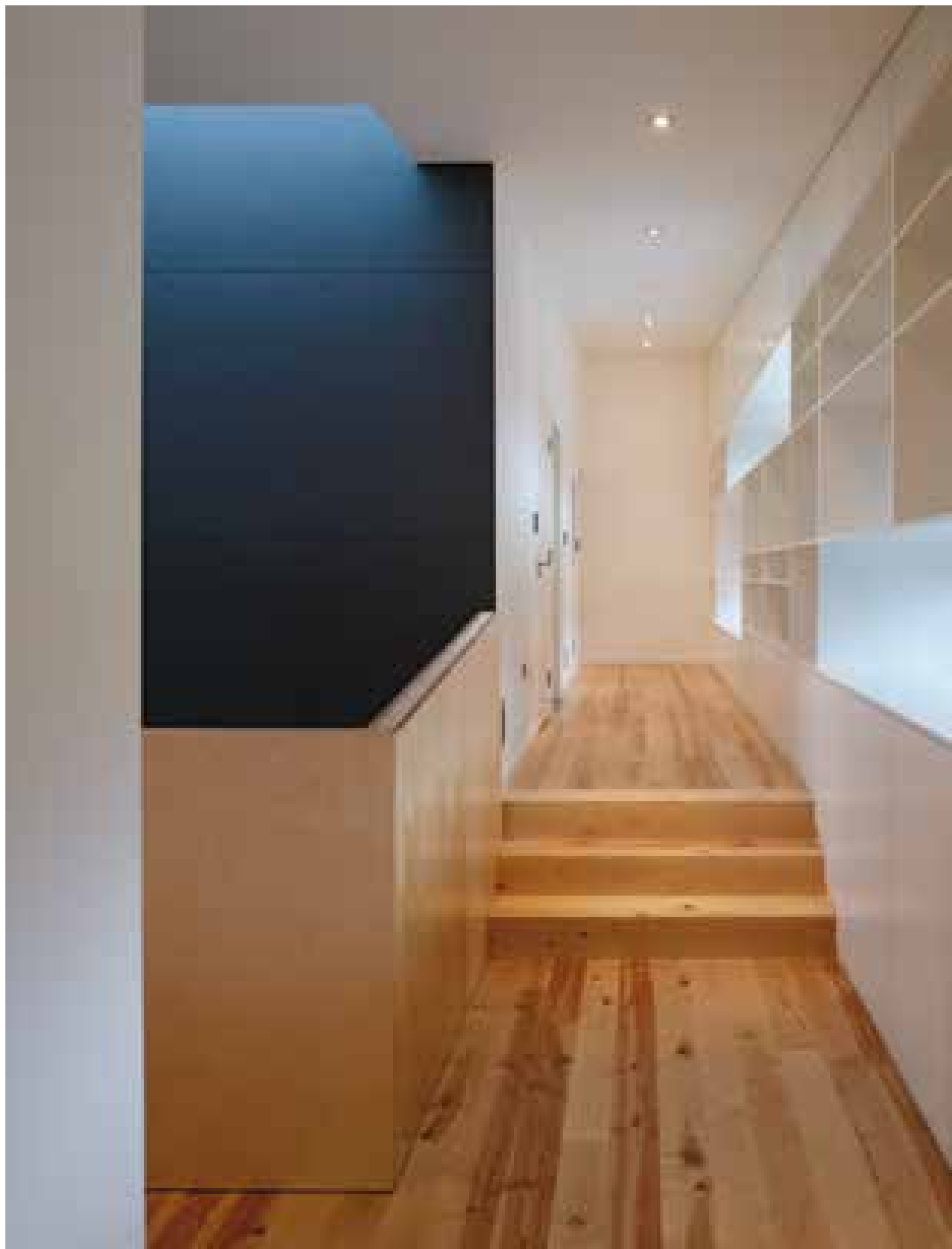
Upper floor, view of the hallway looking south The staircase wall is clad with the same fibre cement panels as the façades.
